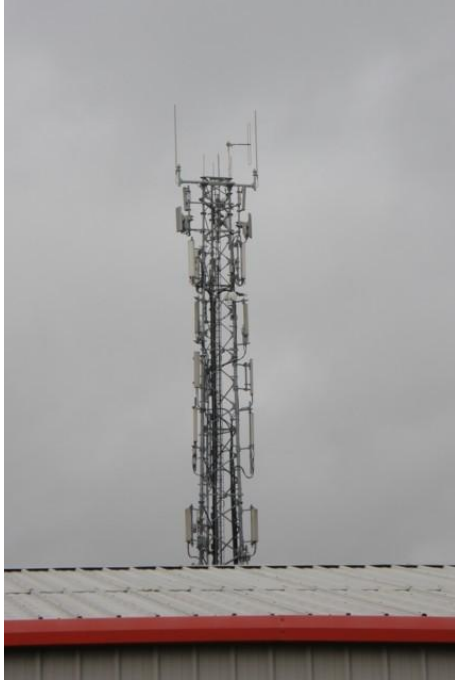
Transmitter Site Photo
